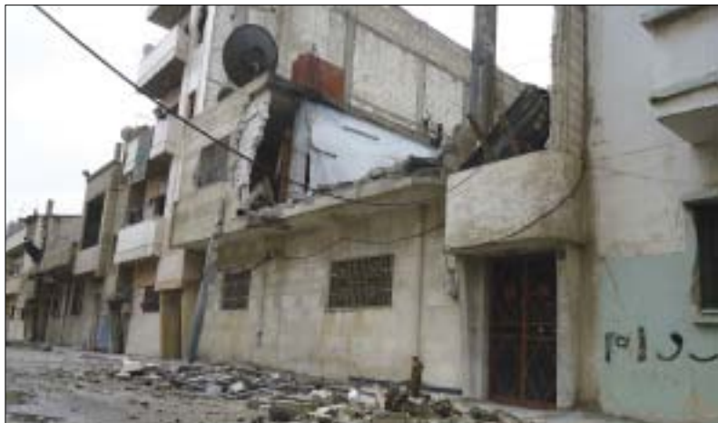
Homes damaged by shelling in Homs, Syria.
