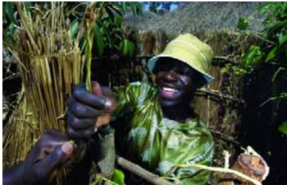
Otii Celcius, a seminary student, helps build the mud brick wall of a new latrine in Awer camp for internally displaced persons near Gulu, Uganda, in 2004. The seminarians perform community service in the camps.
