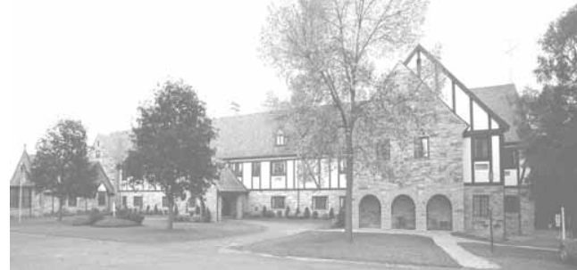
Guest House Men's Treatment Center Rochester, Minnesota
