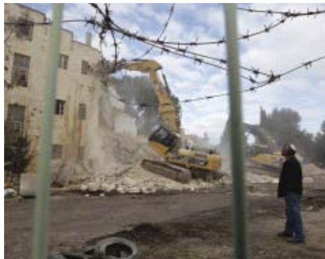
Excavators demolished the Shepherd Hotel in the Sheikh Jarrah neighborhood of East Jerusalem on Jan. 9, clearing the way for 20 new homes for Jews in the contested area.
