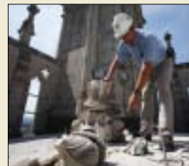
Damage at the National Cathedral
